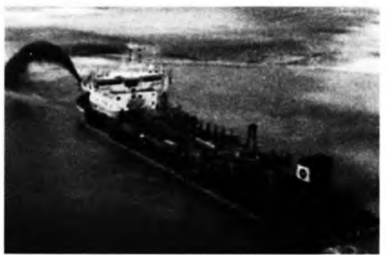
Fig. 25: Dredging for forming the island
