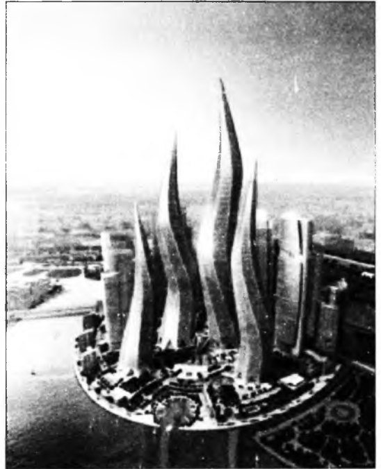
Fig. 18 : Sama Dubai Towers
