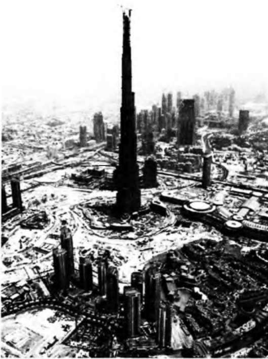
Fig. 13: Burj Dubai under construction.
