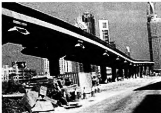
Fig. 11: Metro under construction
